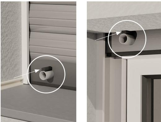
For optimum effectivity, also apply a small strip of soni SOFT-CLOSE to both stoppers (see drawing). This will dampen the impact of the roller shutter when pulled up against its box.
